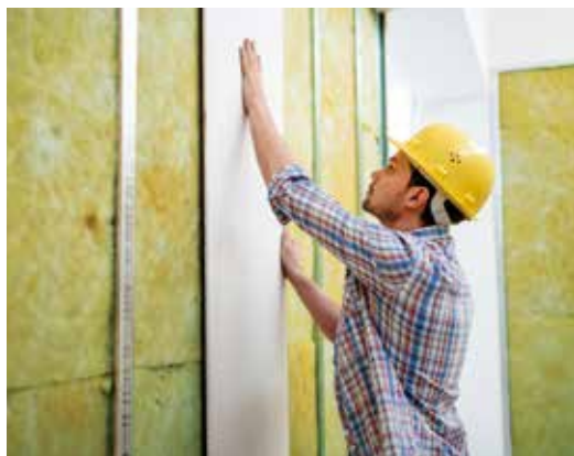
Drywall system installation with stonewall inside and FIBRANgyps plasterboards.
